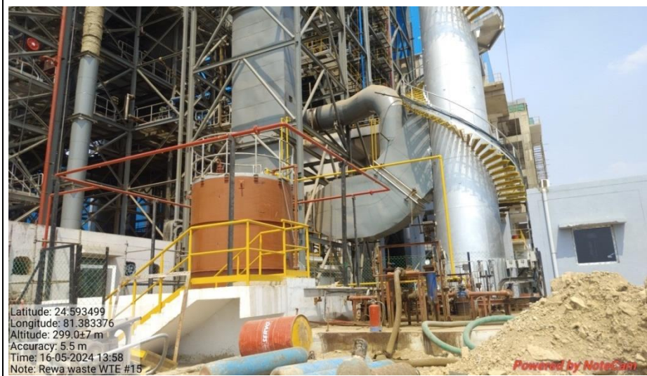
Waste to Energy Plant
