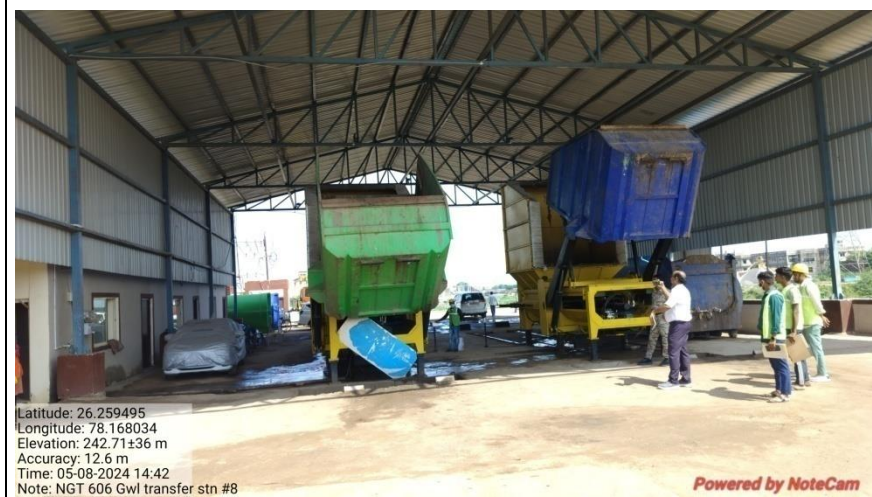
Transfer Station, Jalalpur FCTS
