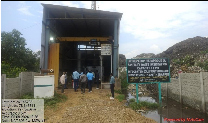
Hazardous & sanitary waste incinerator
