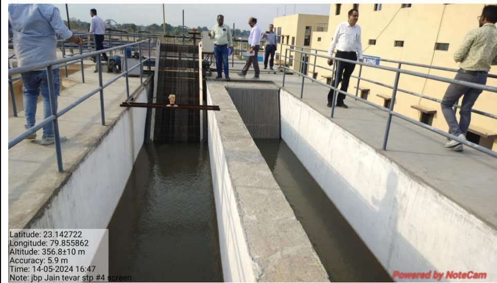
Under trail STP 29 MLD at Tevar
