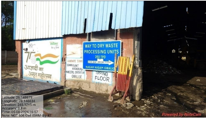
Solid Waste Processing Unit, Kedarpur, Gwalior
