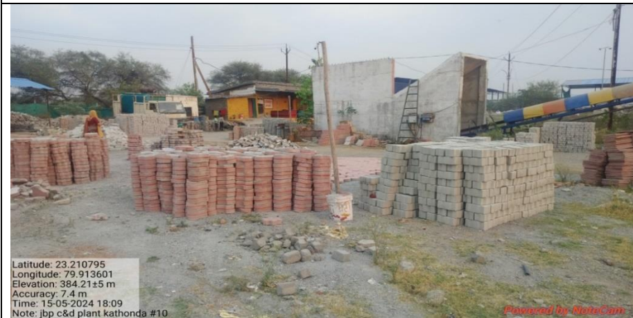
Manufacturing of Paver blocks at C & D waste processing plant
