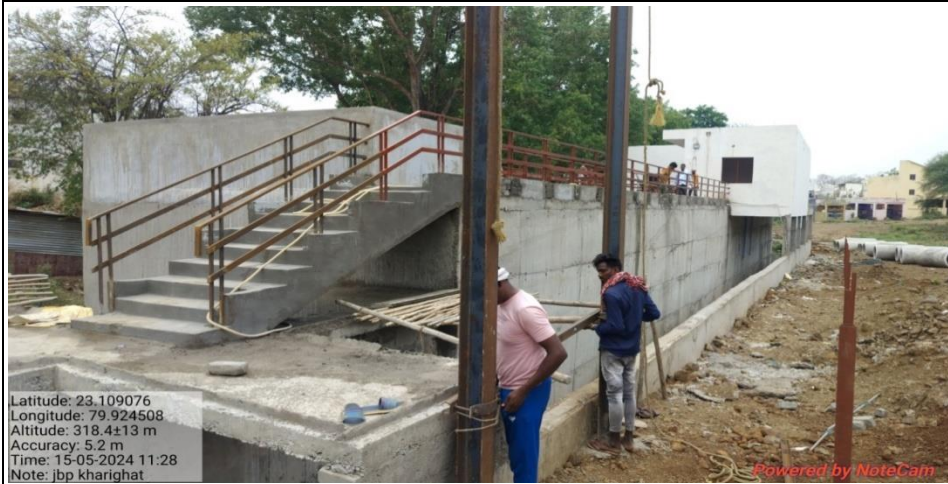
Under construction STP at kharighat
