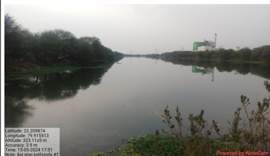
Waste stabilization pond, Kathonda
