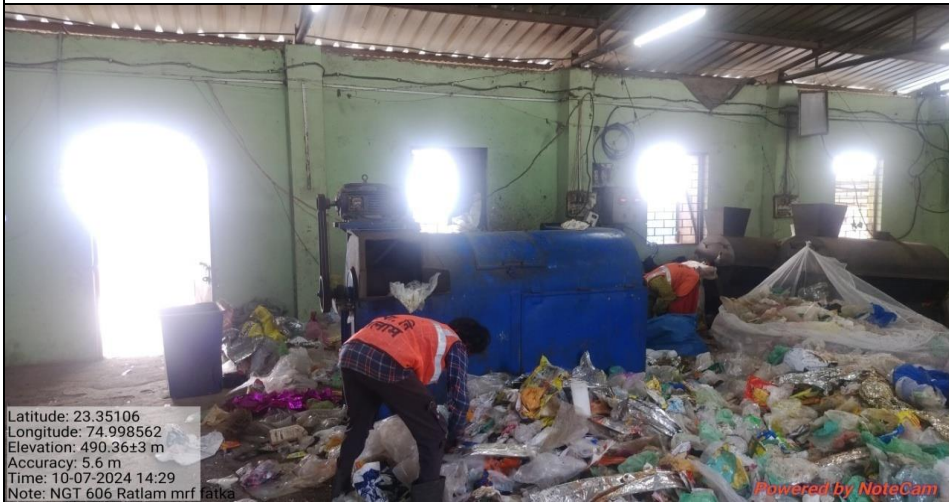
Processing of Plastic waste at Fatka Machine
