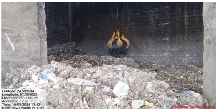
RDF being fed into Waste to Energy plant
