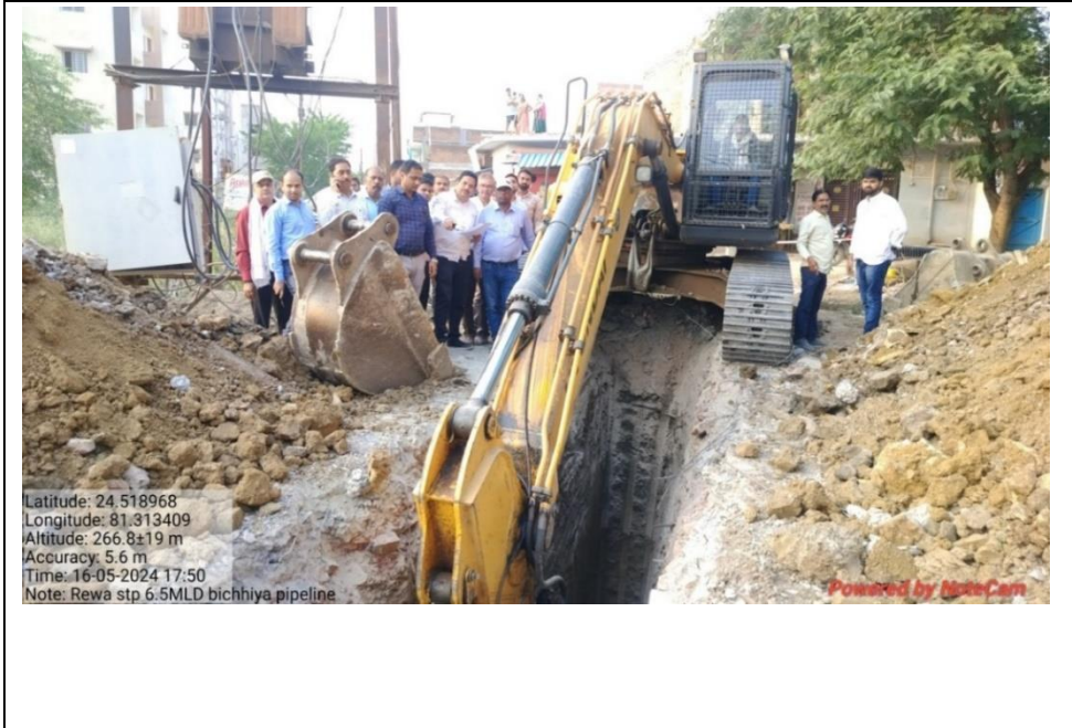
Laying of sewerage network in Rewa city
