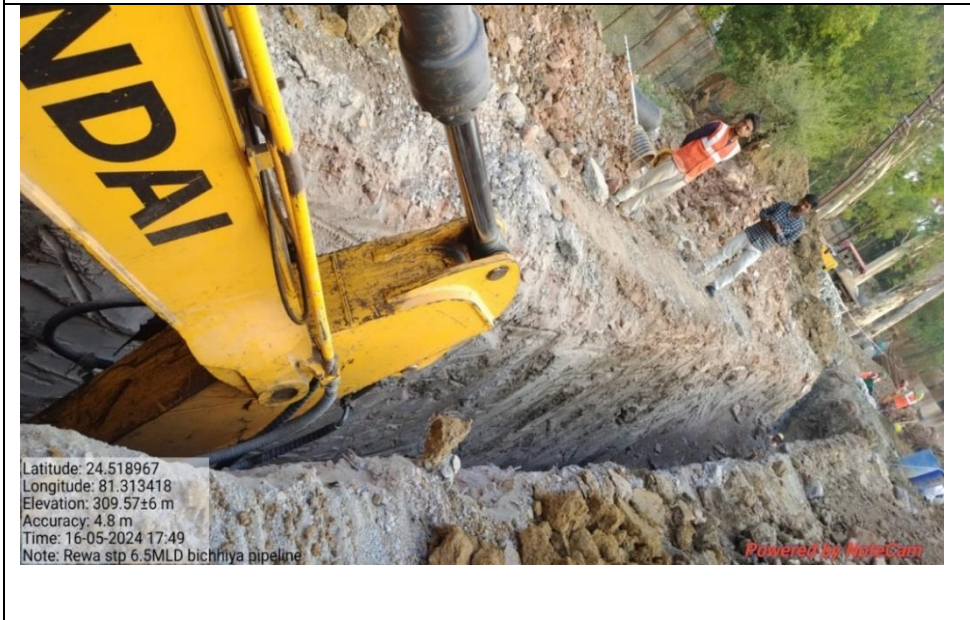
Laying of sewerage network in Rewa city
