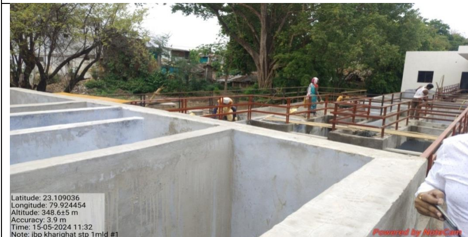
Under construction STP at Kharighat
