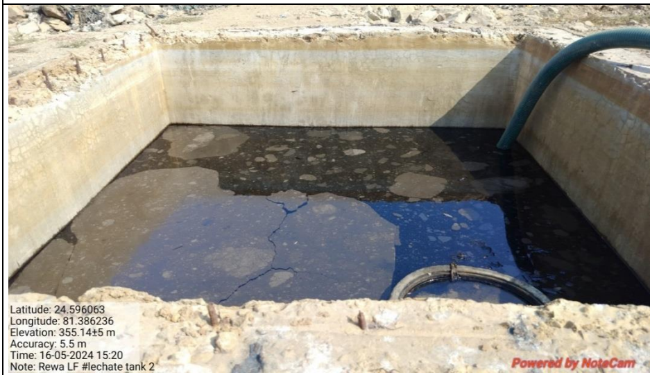
Leachate tank near Sanitary landfill site
