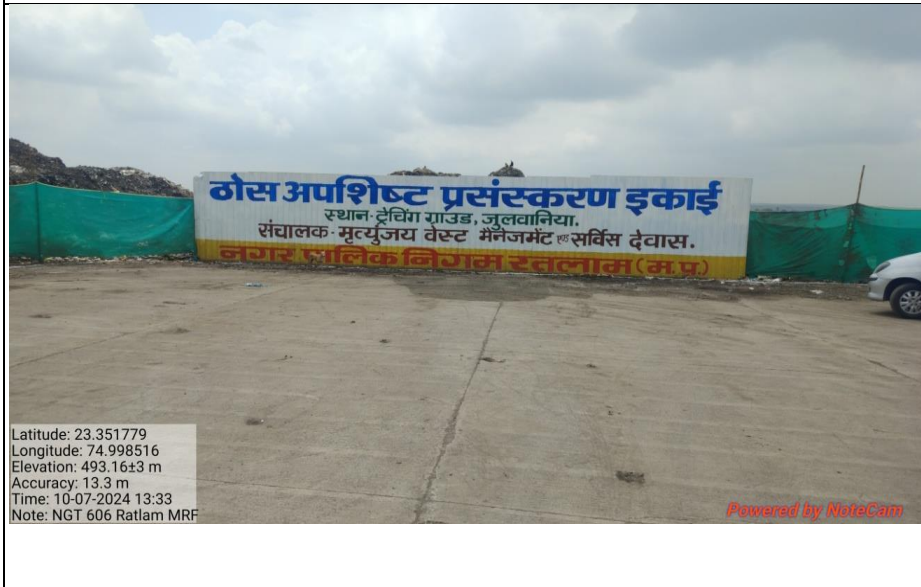
Solid Waste Processing Unit, Julvaniya, Ratlam
