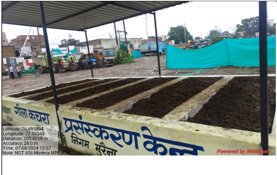
Compost pits at waste processing unit
