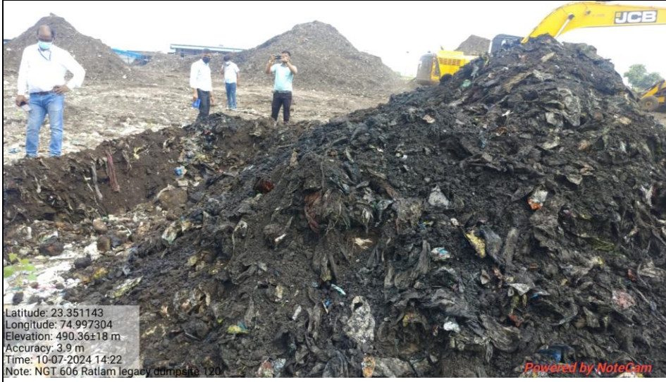
Legacy waste excavated at reclaimed land upto 7-8 ft depth
