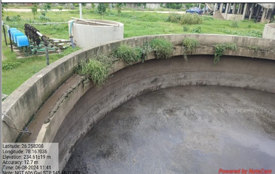
Weeds grown on Sludge thickener
